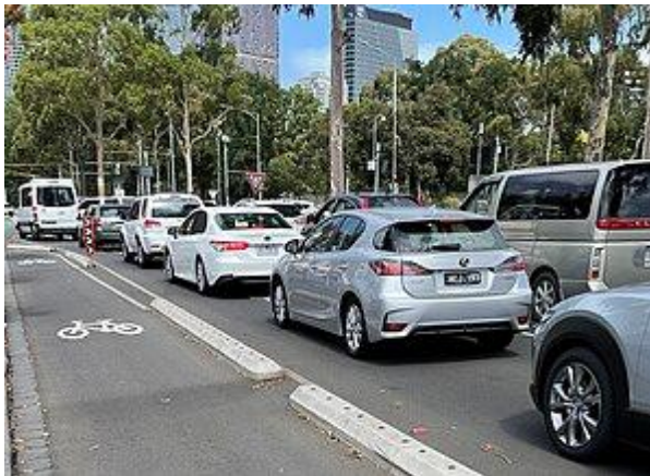
2.3 – Protected bike lane (cycleway)
