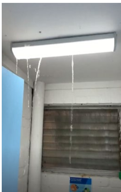
Significant structural issues at Cohealth in Collingwood leads to emergency closures of spaces when roofs leak through lighting fixtures.
