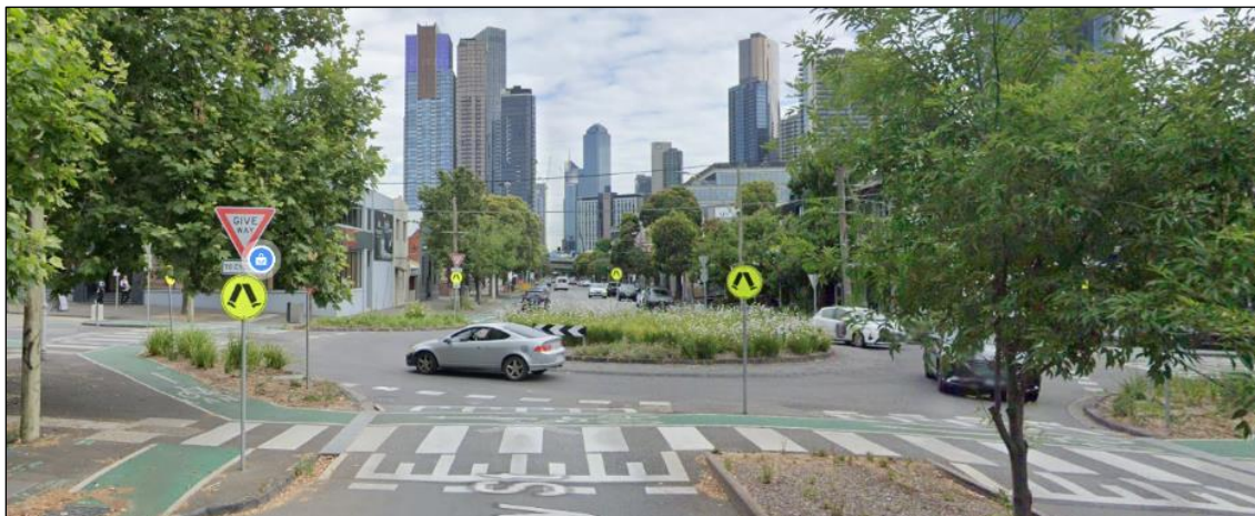
Figure 18 - Example of a protected roundabout
