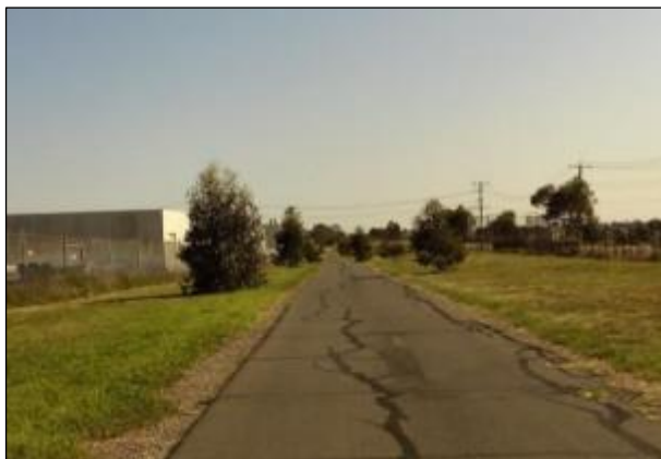
Figure 12 – Example of a shared path with no streetlighting (Federation trail shared path)
