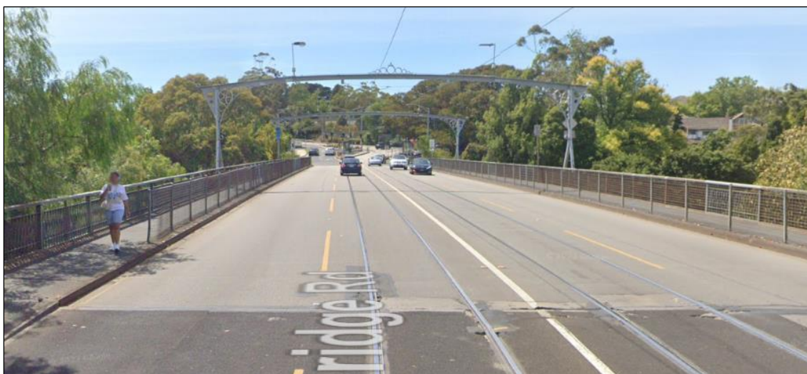
Figure 20 - Example of a bridge that was considered too narrow to provide a separated cycling facility. A separate structure was recommended as a potential solution at this location.
