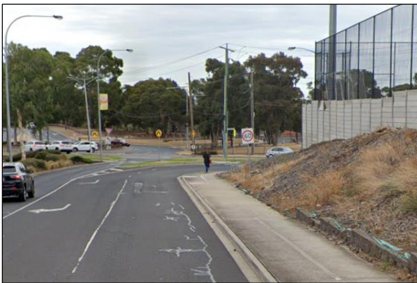
Figure 10 - Example of a two-way separated off-road facility
