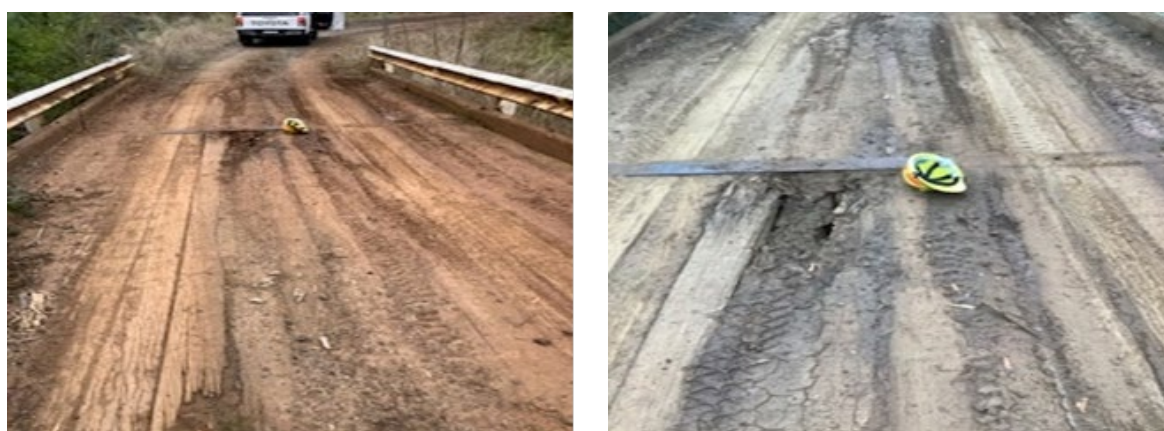
Figure 6 Tanners Road bridge, Calignee South Road, Gippsland
