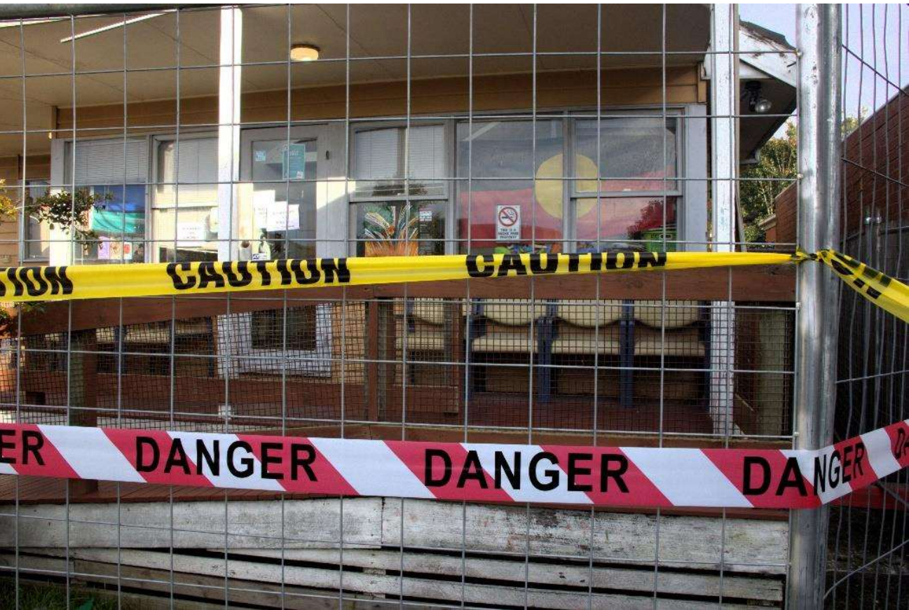
Dandenong and District Aborigines Co-operative Ltd (DDCAL) was forced to close its Stud Road headquarters in August 2024 due to structural failure and the risk of asbestos exposure. Source: Infrastructure Victoria and VACCHO, Investing in Aboriginal health and wellbeing infrastructure .
